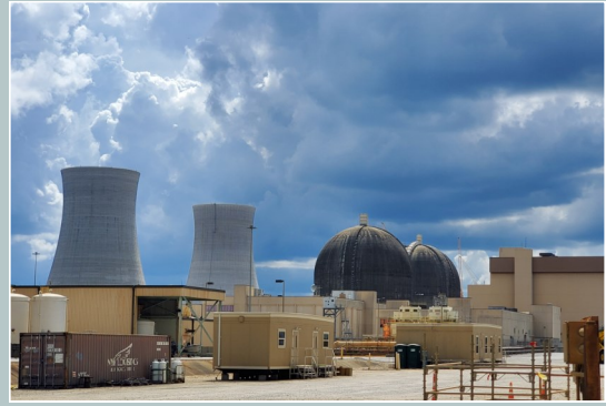
Recent View Showing Construction Trailers (7-21)
